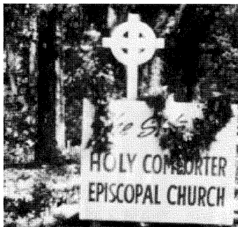
Sign identifying future site of Holy Comforter Episcopal Church on Miccosukee Road
